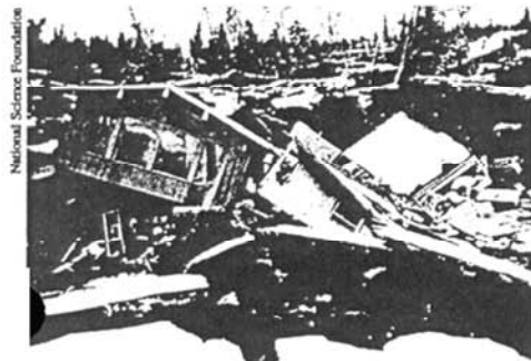
Figure 1.4: House on Turnagain slide
