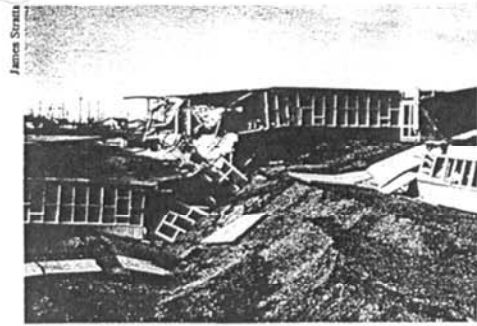
Figure 1.3: School straddling a landslide-induced rupture, Alaska
