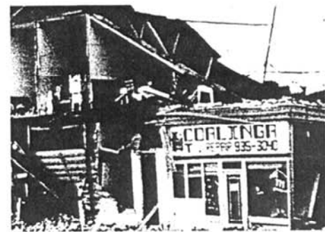
Figure 1.12: Damage to an older masonry building
